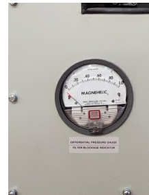
Optional Differential Pressure Gage (Filter Blockage Indicator) available
